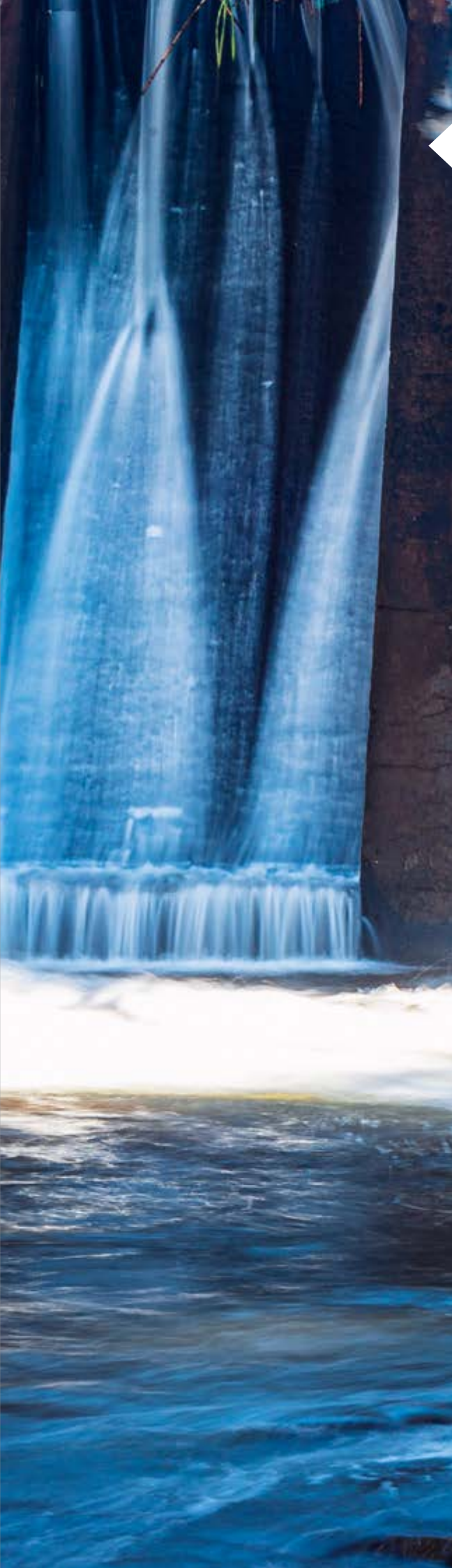
Dam in municipal park, Paraná, Brazil
