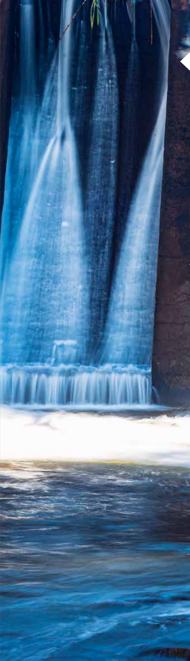
Dam in municipal park, Paraná, Brazil
